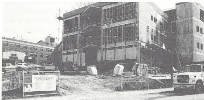
View of Center for Molecular Electronics construction
