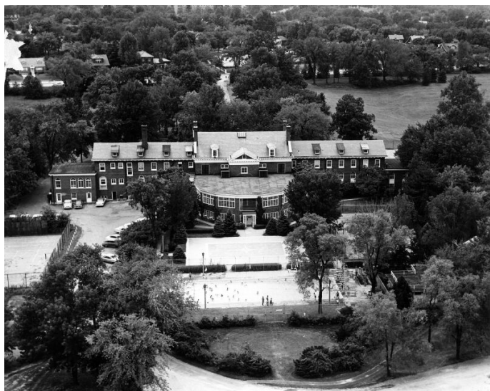
The old administration (Bellerive Country Club) building.
