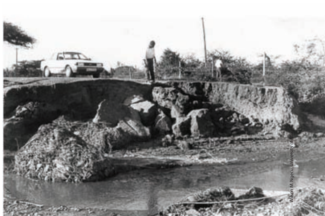
A section of Massii-Makueni high were a major bridge was destroyed by a late 1990s landslide
