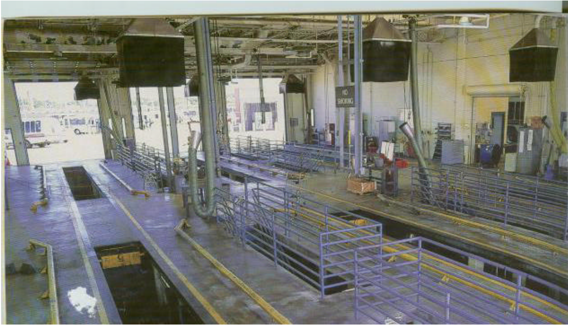
Fig.4. Interconnected Underground Pits
